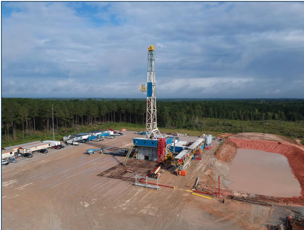
Figure 3: Nabors B14 on the Stewart/Bergold location during rig up
